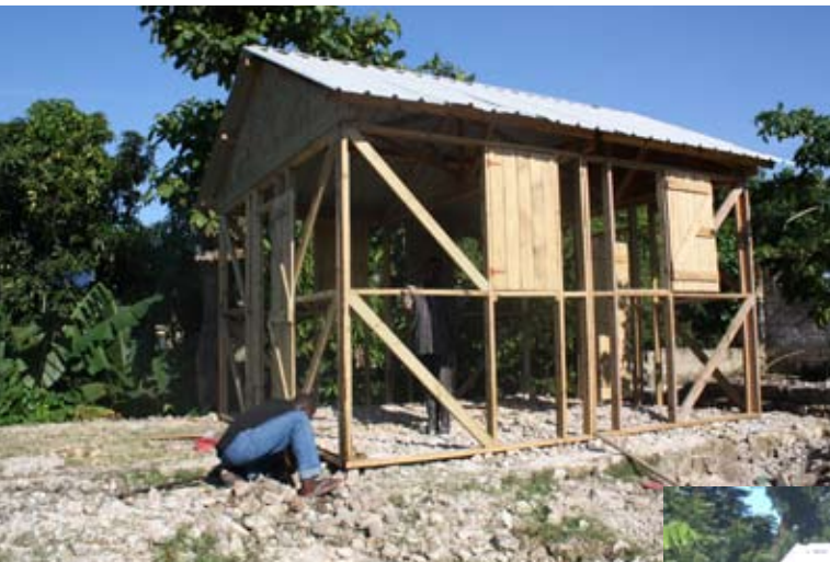
Homes being built after the earthquake in Haiti
