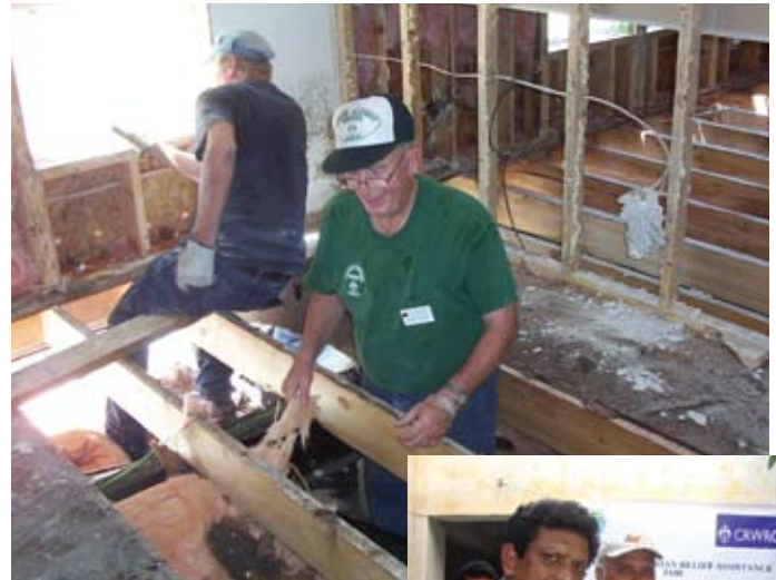
CRWRC volunteer Harry Faber (green shirt) works alongside a local volunteer to gut a flood-damaged home in Colfax, Iowa.
