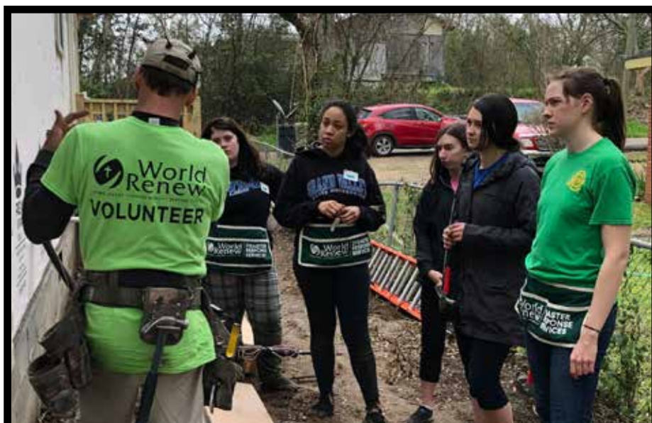
Dave, a volunteer from Orland Park CRC, teaches GVSU students how to install siding.
