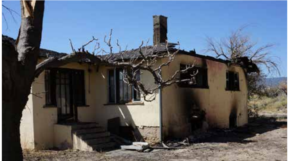
Former main parsonage of Naschitti CRC, destroyed by fire Aug. 20, 2019.
