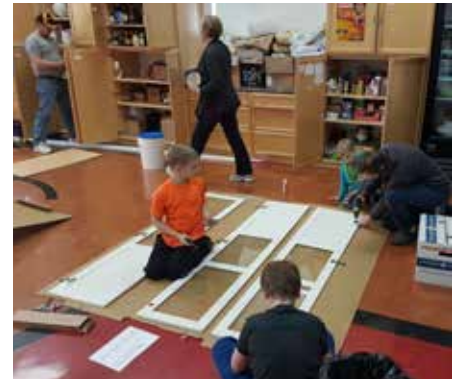
Boys and leaders from Covenant CRC's Cadet club help construct new cupboards at the Indigenous Family Centre in Winnipeg, Man.
