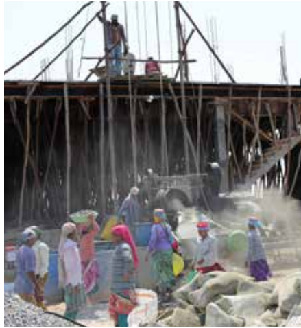
New Hope Children's Home under construction, Oct. 2018.
