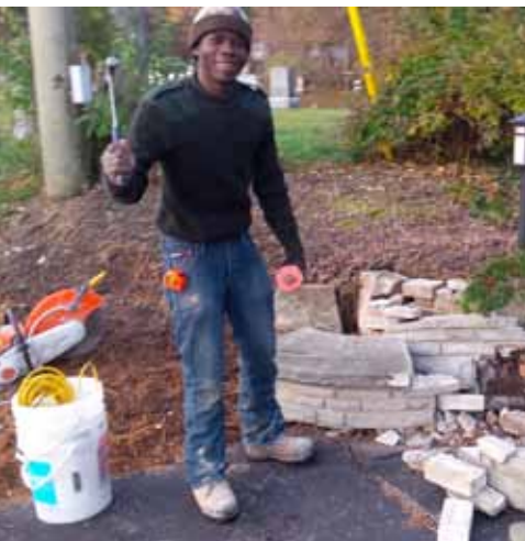
Mwana Hardy of Just Working Construction works on a job site.
