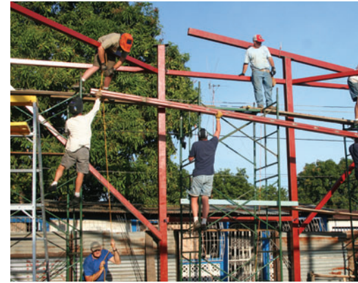
Volunteers from DeMotte, Ind., construct a church Managua, Nicaragua.
