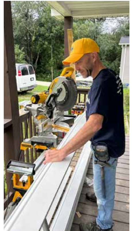
Eric Bolt from Messiah Christian Reformed Church in Hudsonville, Mich., cuts trim at a work site in Hendersonville, N.C.
