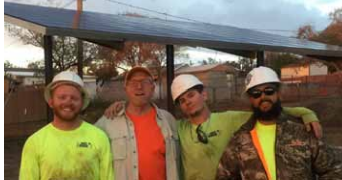
Rick Kruis (orange shirt) with the crew that installed Bethany CRC’s solar carport.
