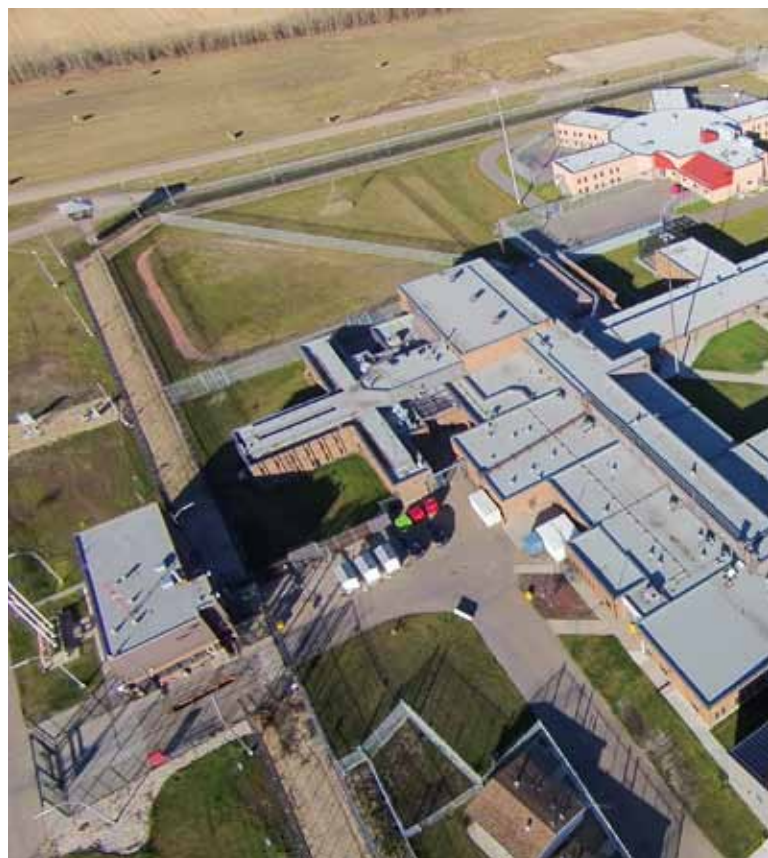
Edmonton Institution, Correction Services Canada's maximum security facility in Edmonton, Alta.
