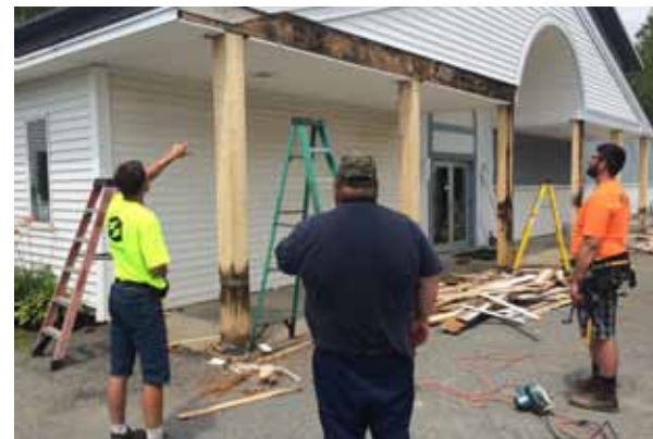
Repairs at Penobscot Christian School.
