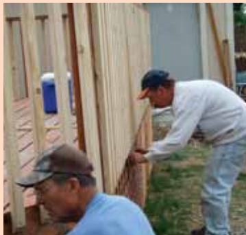
Volunteers help repair a deck.
