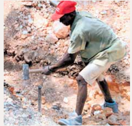
Digging the foundation for Jacquet CRC’s new building.
